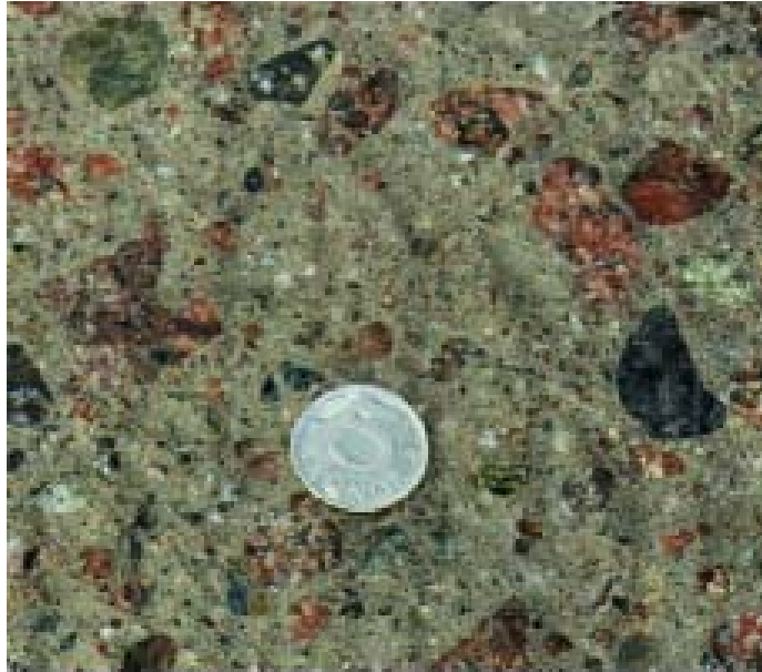
Figure 4. After cleaning with high pressure water.
