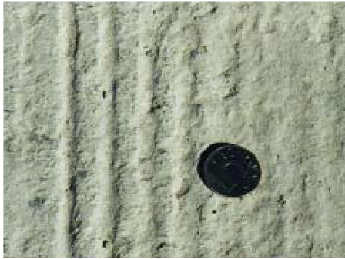
Figure 3. Surface after milling
