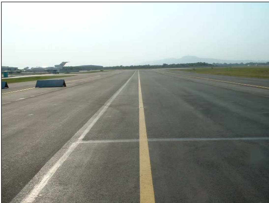
Figure 2: CTI Airport Taxiways Longitudinal Joint Surface Sealing
