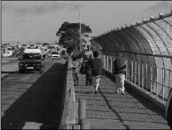
Photograph 5: Cage on road bridge
