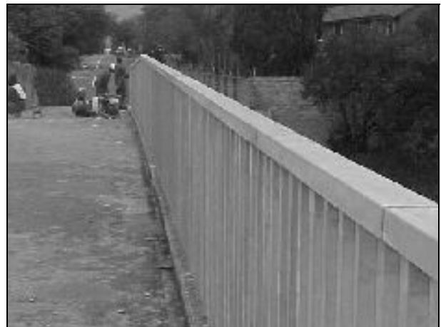
Photograph 5: New pedestrian rails
