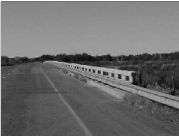
Photograph 4: New concrete handrails
