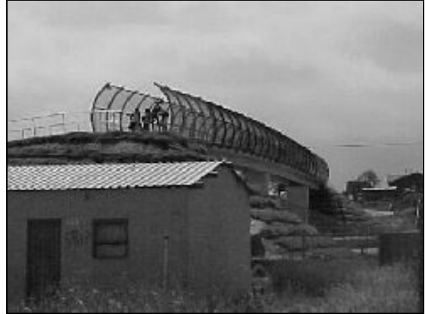
Photograph 6: Caged pedestrian bridge
