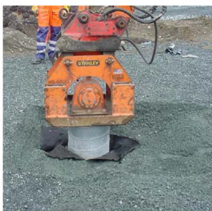
Figure 3. – Installing steel tube
