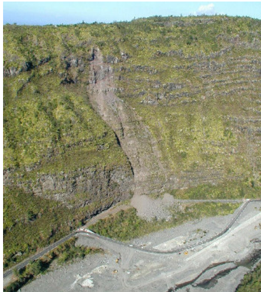
Figure 8 : Avoidance of an active crumbling of 10 000 m 3 (R.N. 5, road of Cilaos)
