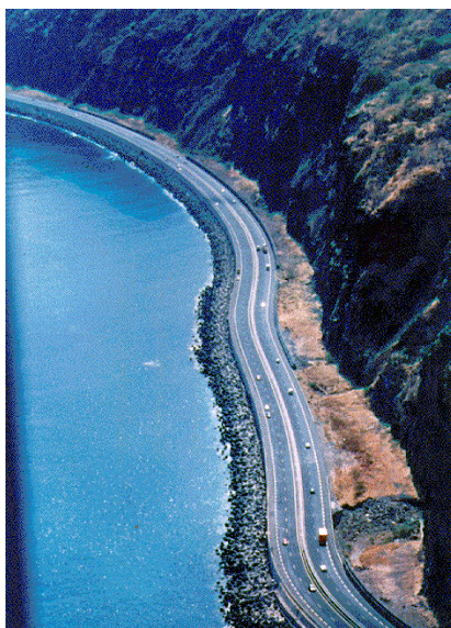
Figure 3 - Air sight of the road of the littoral
