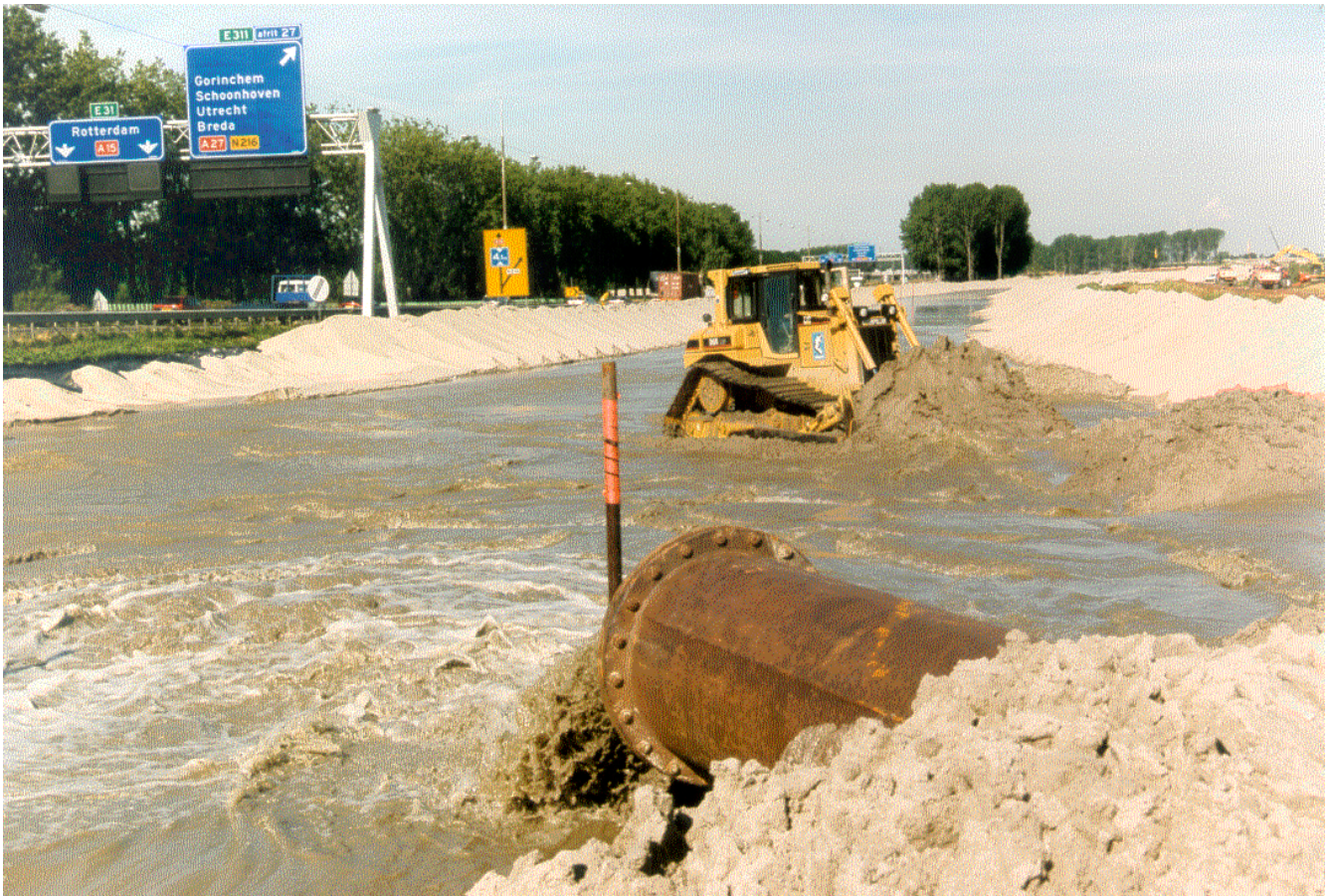
Figure 2 - A-15/E-31 motorway and Betuweroute under construction
