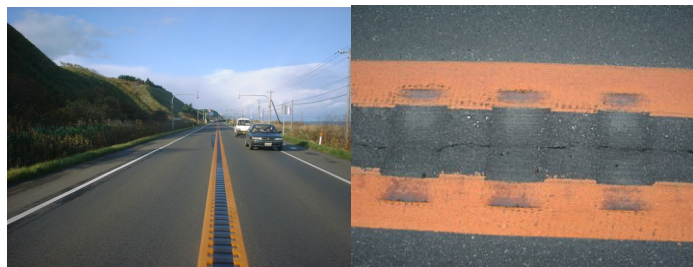
Photo 3 Rumble strips in service
