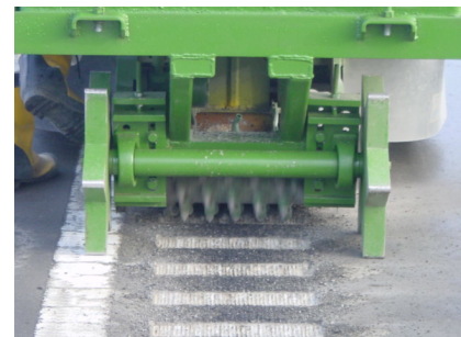
Photo 4 Milling of narrow grooves
