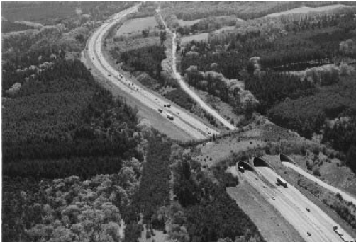
Fig. 2 - A landscape bridge (Photo by Luchtfotografie Slagboom en Peeters) and an underpass (Photo by B. Iuell)
