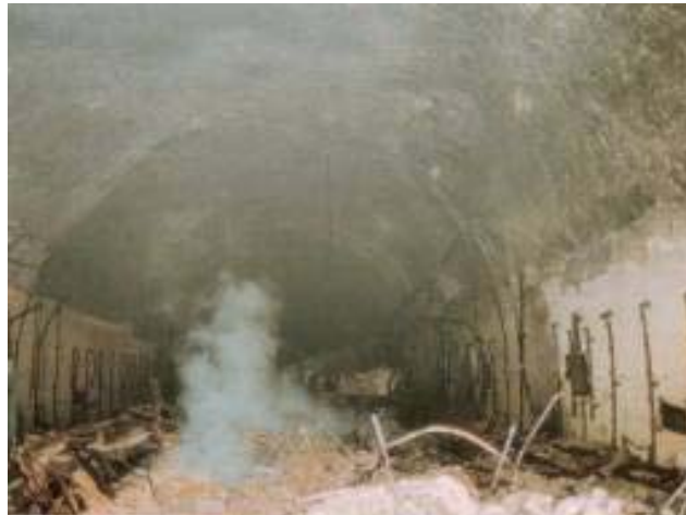
Figure 2. Nihonzaka Tunnel fire accident
