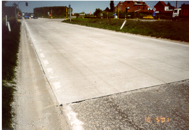
Figure 8: Appearance of the UTW pavement
