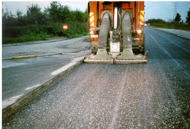
Figure 3: Cleaning the planed surface under pressure
