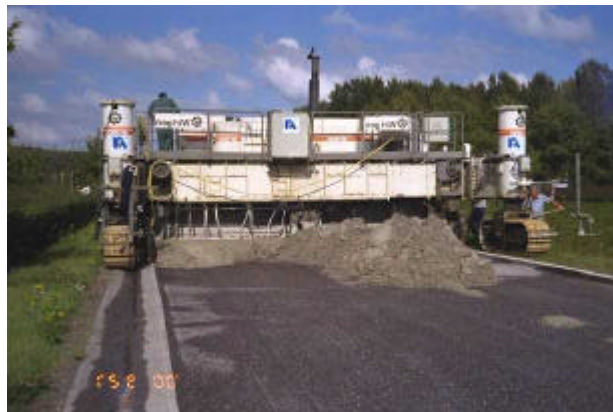
Figure 6: Production with a slipformpaver
