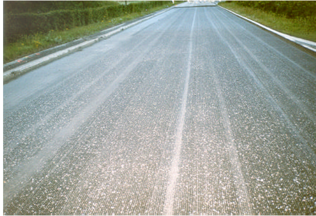
Figure 2: Flat-milled asphalt surface
