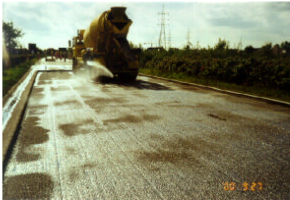
Figure 5: Dampening the asphalt surface just before concreting
