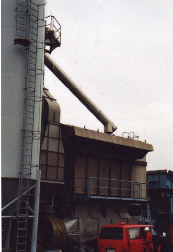
Figure 5 CO 2 Measurement at the plant
