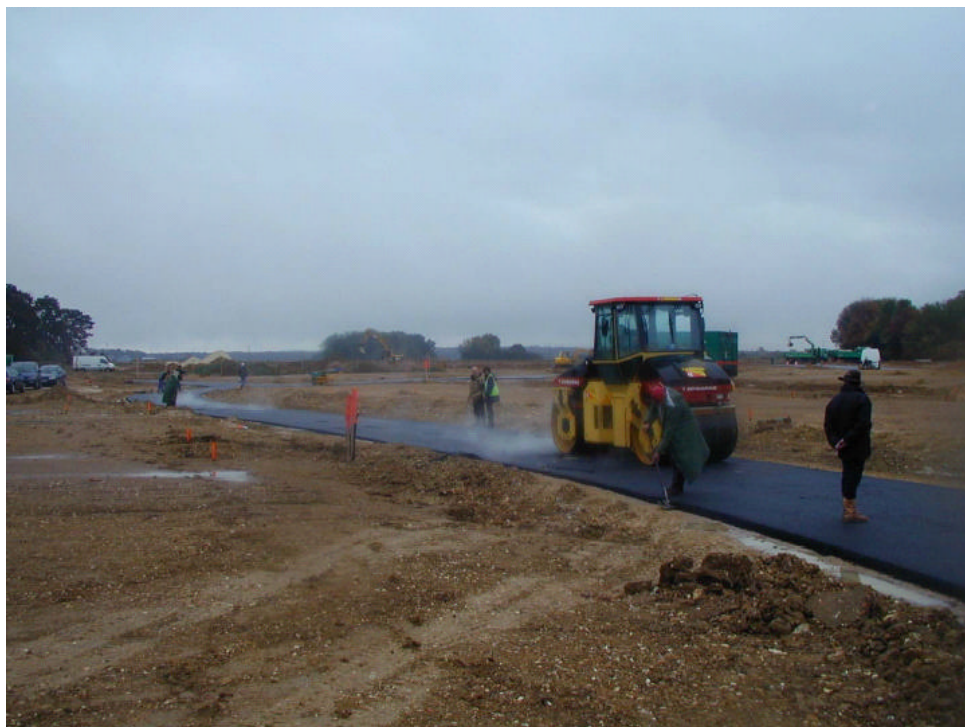
Figure 8 Application and compaction of AC with aspha-min® at 120 °C in France
