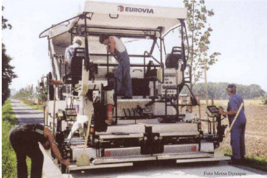
Figure 1 Construction site with AC 0/11 + aspha-min®
