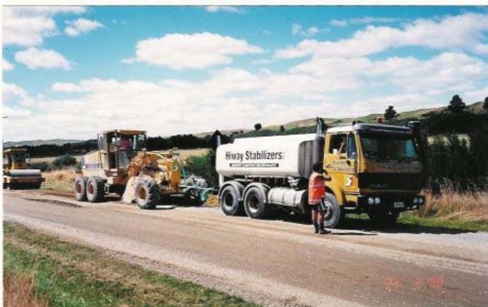
Figure 5 – Recycling Operation (Cement Application, Milling and Primary Compaction)
