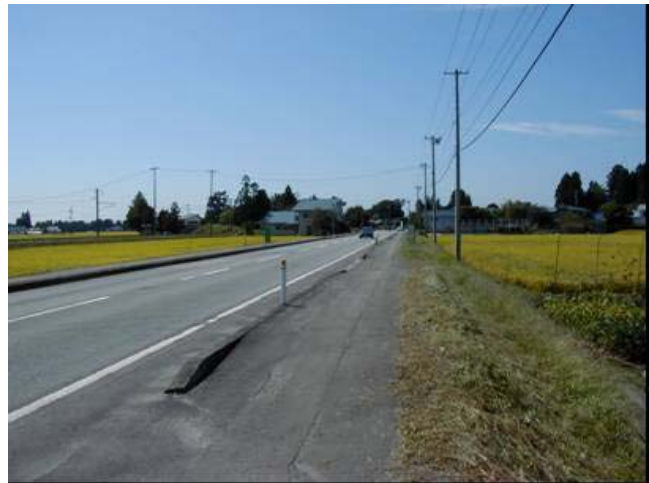
Figure 10 - First test construction site
