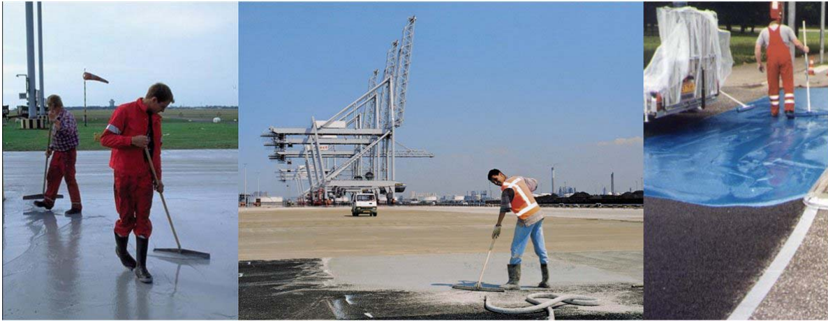
Figure 4 Spreading of micro silica mortar on open graded asphalt, (Densit A/S, 2000).
