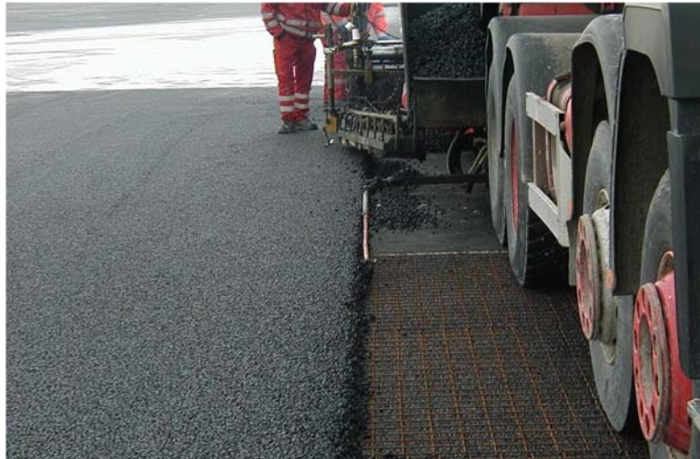
Figure 3 Laying of open graded asphalt on steel reinforcement net
