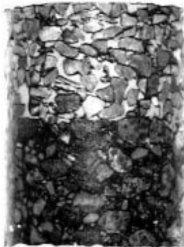
Figure 1 Core of semi-flexible pavement material with bituminous binder course.
