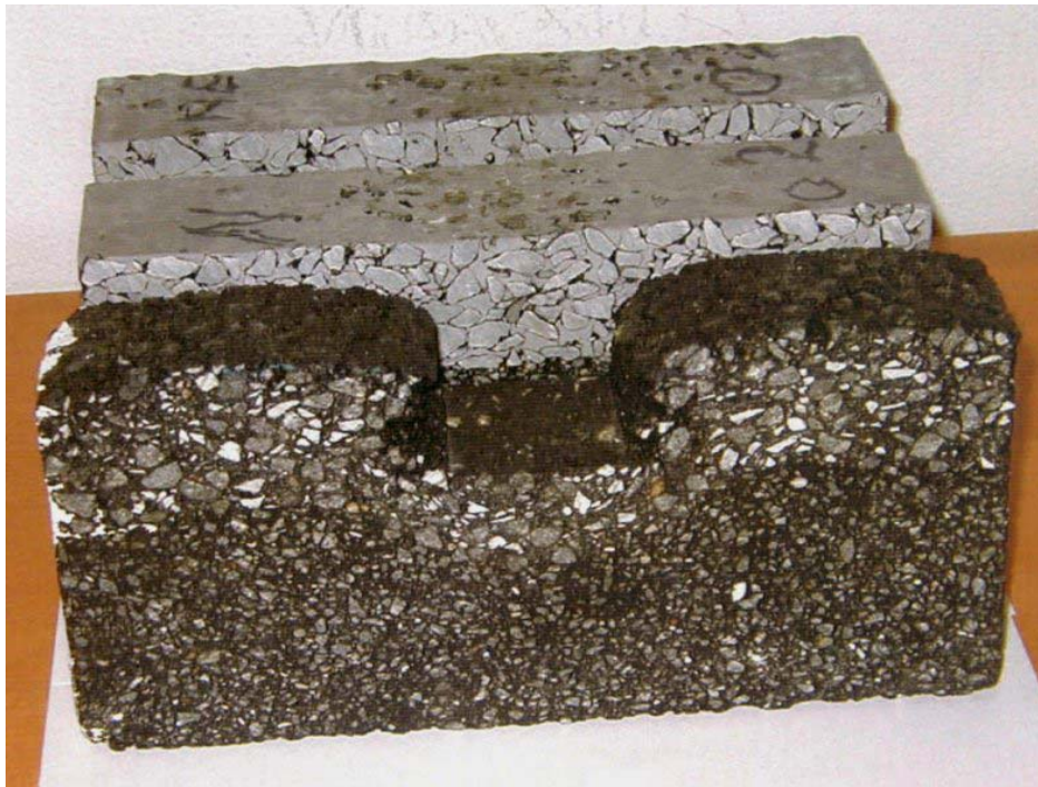
Figure 7 Comparison of the three different pavement structures at the end of testing. In the front is the asphalt wearing course, in the middle the semi-flexible wearing course without steel reinforcement and in the back the semi-flexible wearing course with steel reinforcement.
