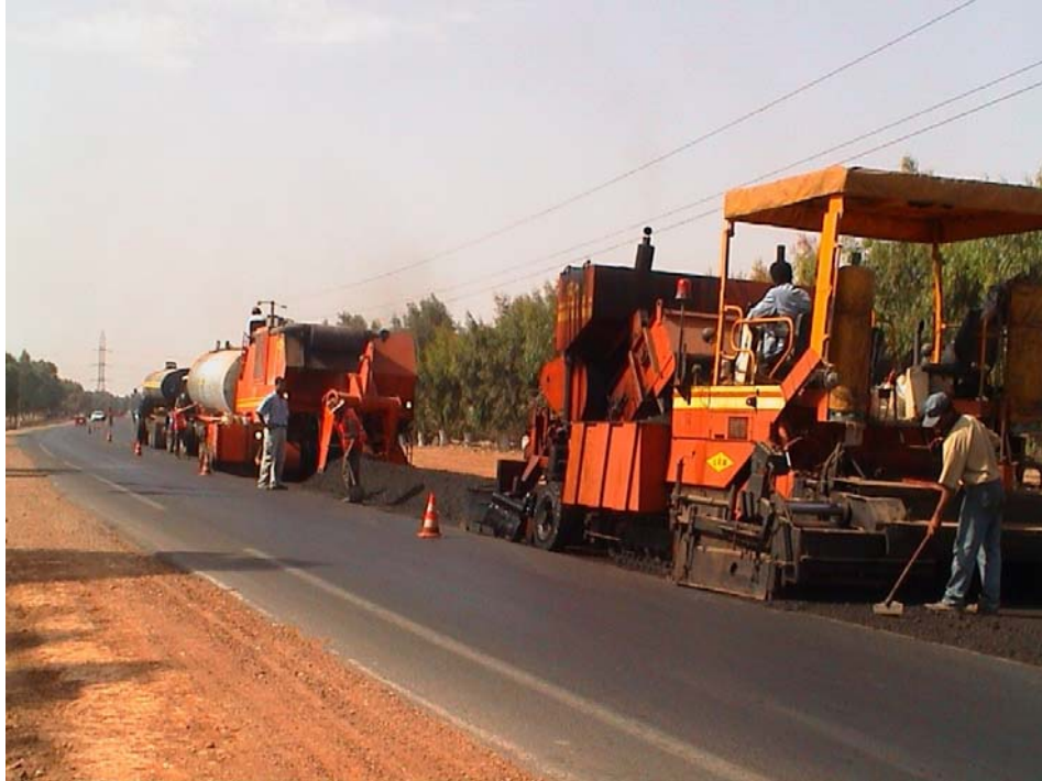
Figure 3 – NOVACOL on-site retreading plant (COLAS)
