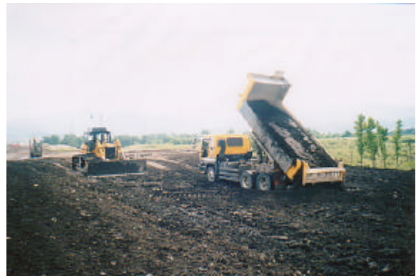
Photo-3 Construction of an embankment using waste casting sand
