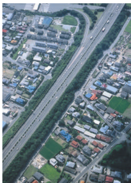
Photo-5 Slopes with forestation
