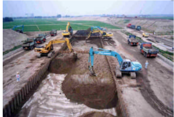
Photo-2 Yard for mixing by-product soils
