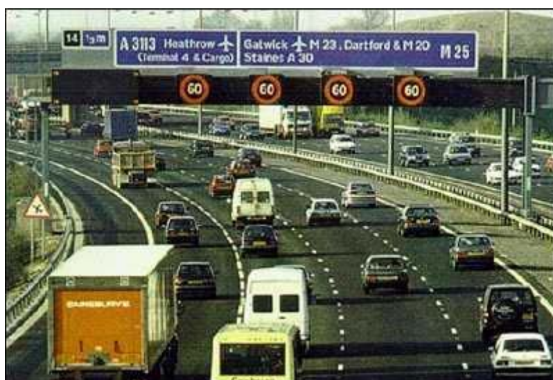
Figure 7: Variable Speed Limits on the M25, London, UK
