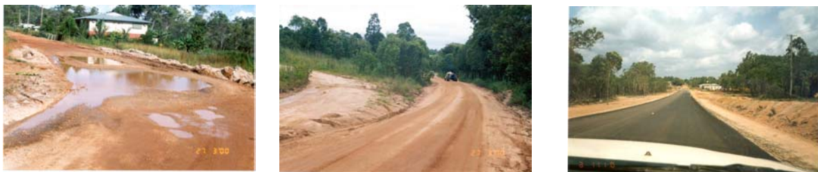
Figure 8. Unconstructed road: wet season and dry season; road following construction
