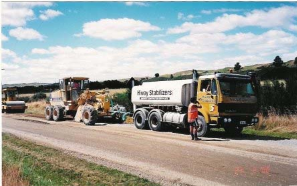
Figure 5 – Recyclage (Application du ciment, fraisage et compactage principal)
