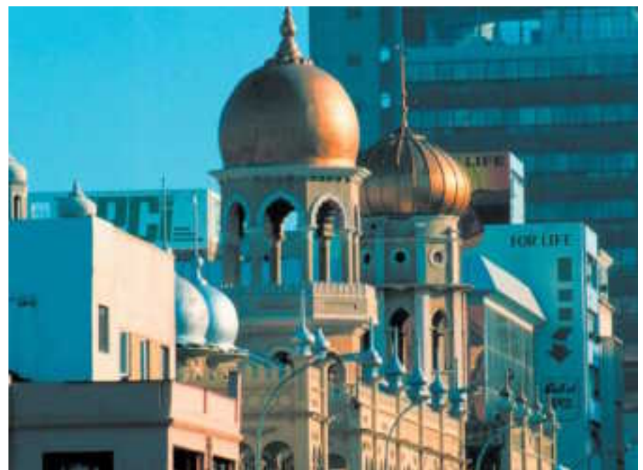
The Grey Street Mosque - an ornate building, the largest mosque in the Southern Hemisphere
